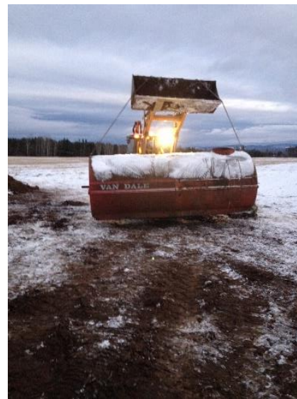
Installation of the deadstock disposal vessel Thunder Bay, ON
