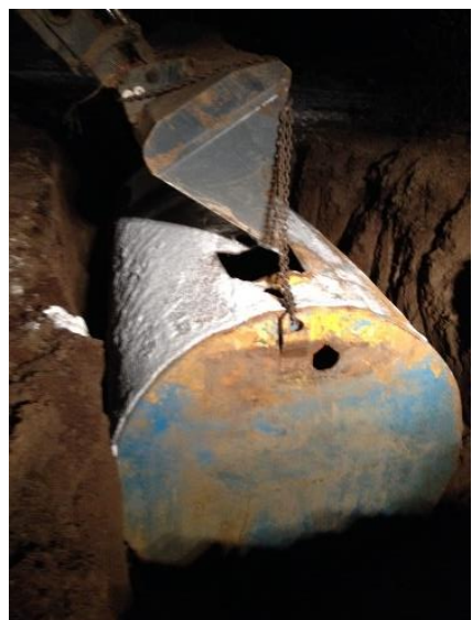
Installation of the deadstock disposal vessel Thunder Bay, ON
